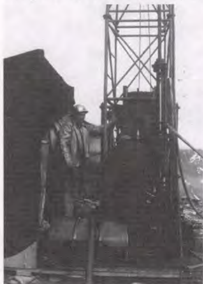
Pulling the core barrel — Sprague and Henwood driller, Joe Elder used wire line to lift core barrel, Sun Deposit, 1977.
