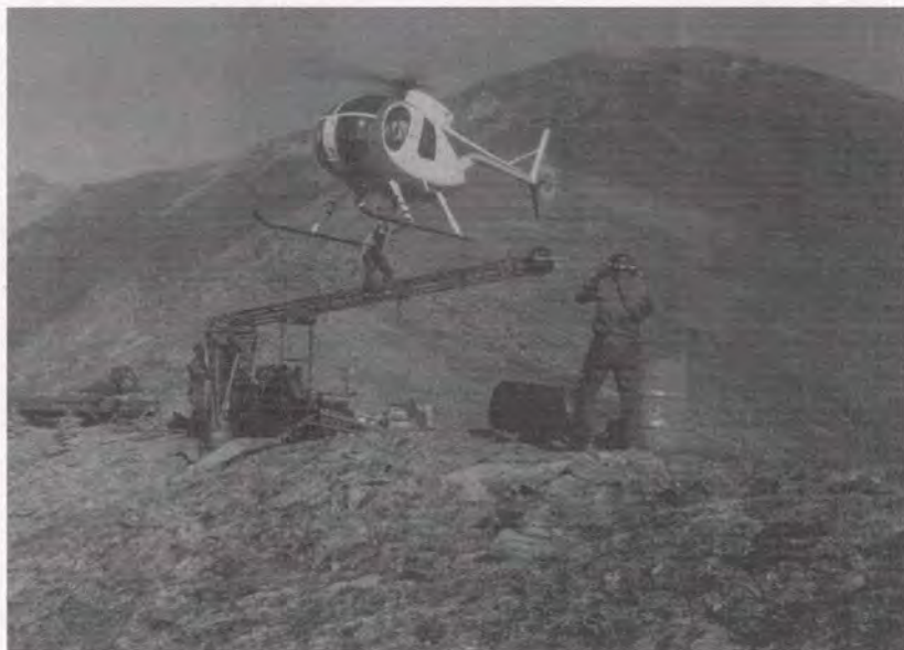
Setting the tower: a Hughes 500c helicopter delicately inches the drill tower into position. Helicopter supported drilling allowed the Ambler deposits to be prospected with little surface disturbance.
