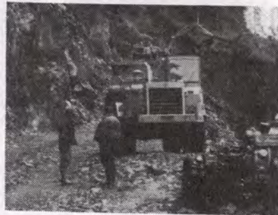
Road construction through tough terrain in May, 1983
